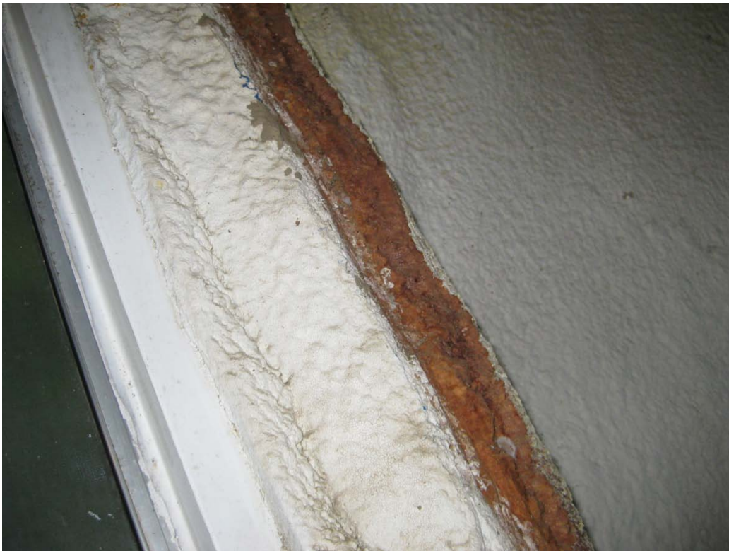
Picture 15: Exposed Foam 1
