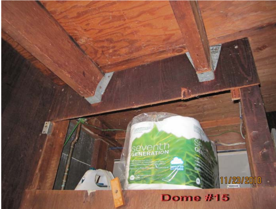
S-1: Dome #15, Condition A, at the hot water heater closet.
