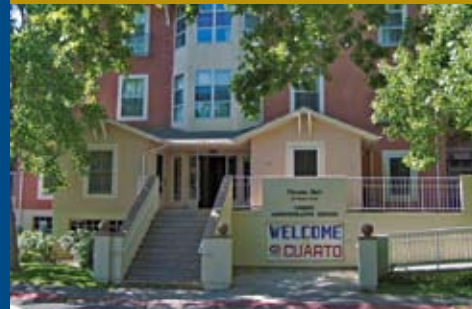
The Cuarto AAC is near the Area Service Desk in Thorson Hall
